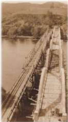
Below: The old bridge collapsed 1929 (centre). Left: two bridges side by side, the old bridge propped up for careful use and to help construct new bridge. Right: New bowstring bridge opened 1933.
