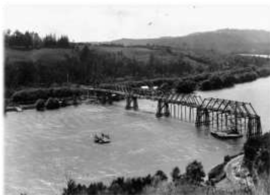
Below: The old bridge collapsed 1929 (centre). Left: two bridges side by side, the old bridge propped up for careful use and to help construct new bridge. Right: New bowstring bridge opened 1933.
